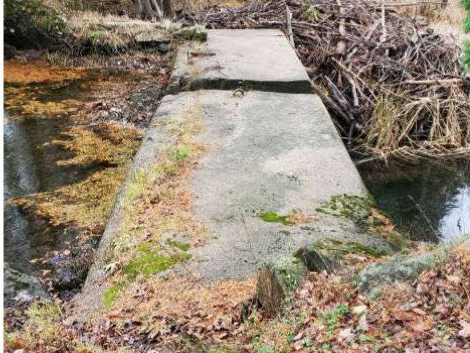
PHOTO#3 – Top of Dam (looking East)
