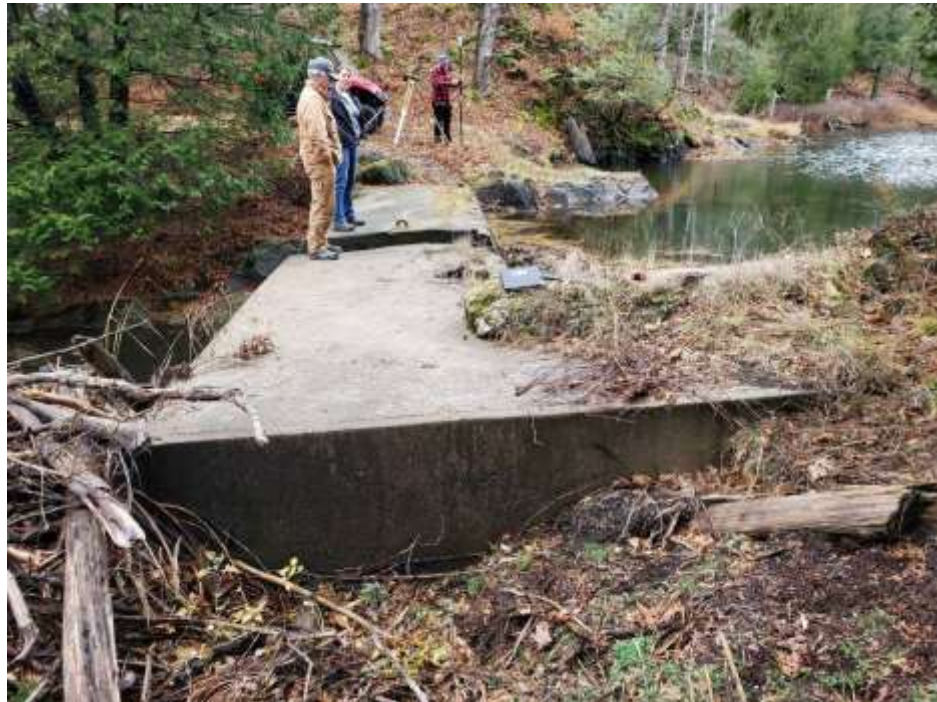
PHOTO#4 – Top of Dam (looking West)
