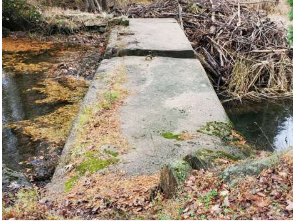
PHOTO#3 – Top of Dam (looking East)
